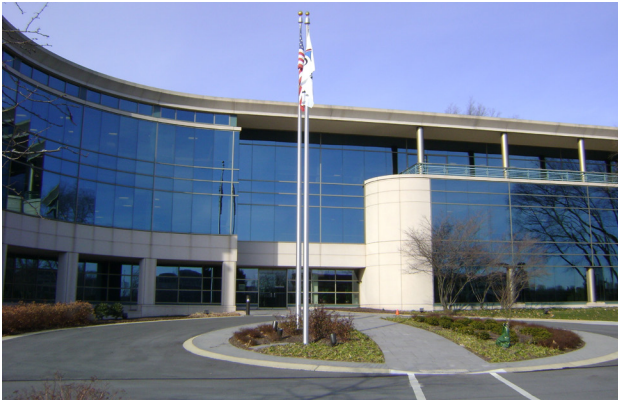
Citadel Federal Credit Union Headquarters in Exton PA
