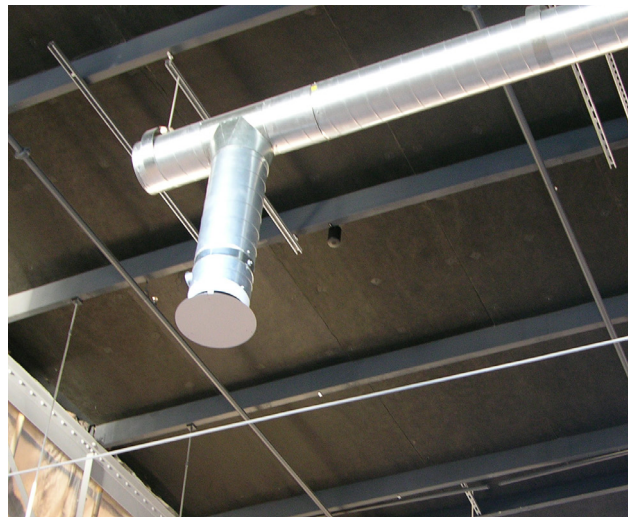
The SGH open office area features areas with 24' ceilings and exposed steel beams (above). The Qt Quiet Technology sound masking system inconspicuously is installed on the exposed beams (below).
