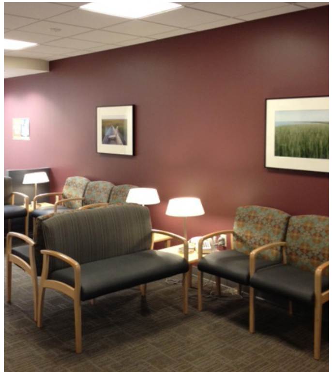
Dover Family Practice Qt 600 Sound Masking Installation
