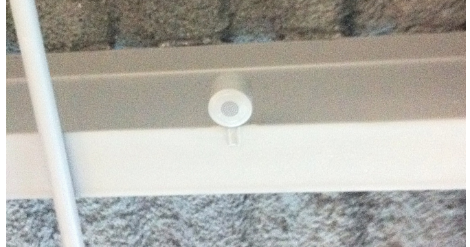
Qt emitter mounted onto an exposed steel beam in the open office area
